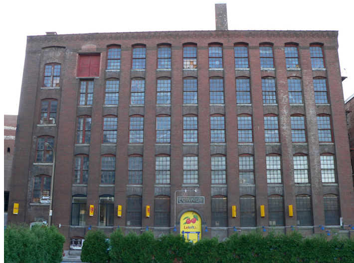
Figure 5. Industrial Building South View: 6-Story Masonry Structure with Wood Floors
